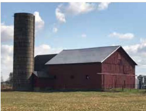
Photo 3 - Simons 1847 Farm Barn
